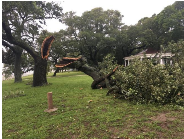
Fallen tree in the front of the mansion June 20, 2017 from Tropical Storm Cindy tornado water spout.
